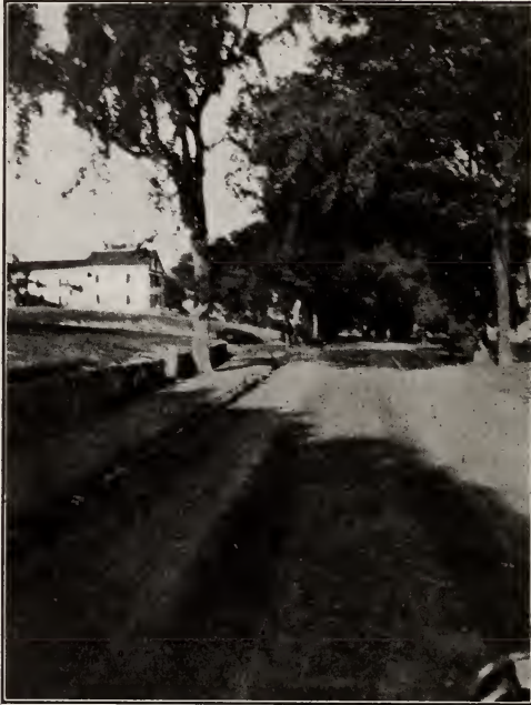
East Street: Failure to Provide an Adequate Thoroughfare Means Today Sacrifice of Fine Trees in East Street Widening
